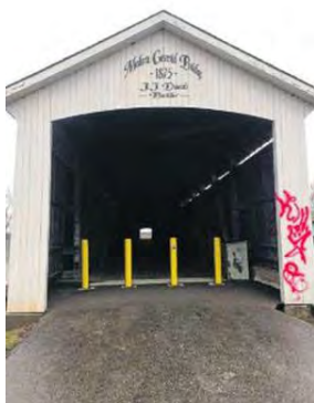
Graffiti is pictured on the western entrance of the Medora Covered Bridge. It's one of about a half dozen spots vandals painted around Dec. 30.
