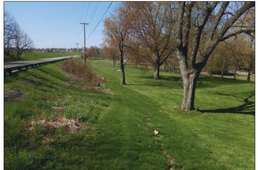
Photo 28: Roadside embankment to the west of S.R. 9, facing southwest.
