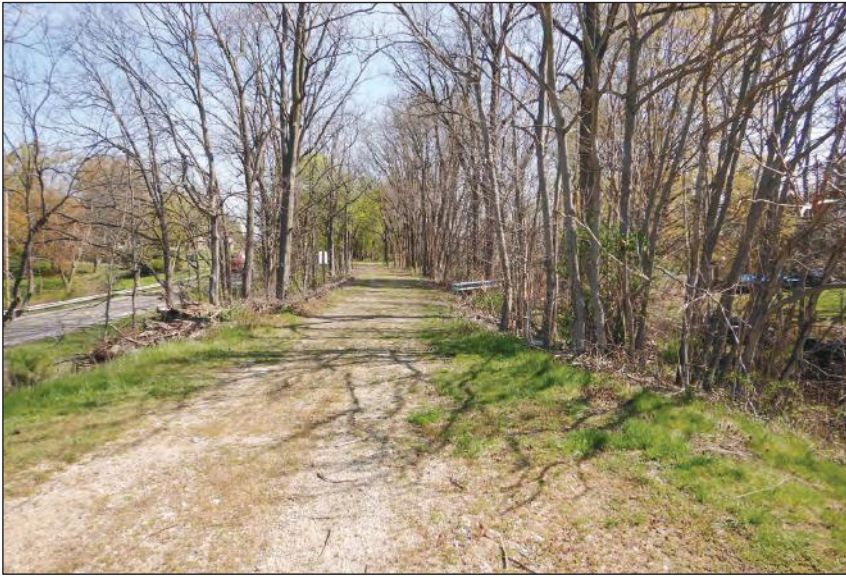
Photo 25: Access road along top of earthen dam, facing northeast.
