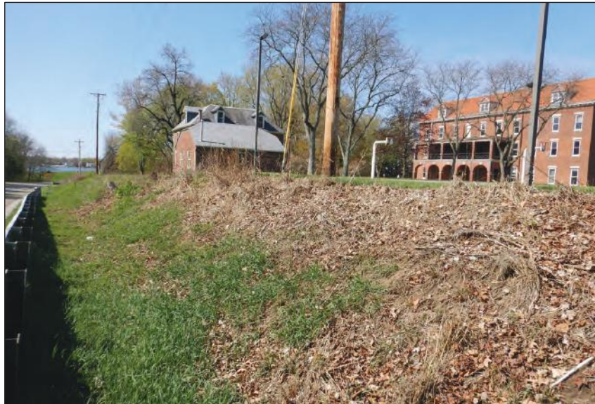
Photo 31: Roadside embankment to the west of S.R. 9, facing southwest.
