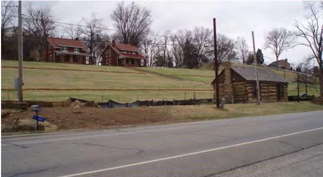
Figure 146. Newburgh Landslide Post Mitigation
